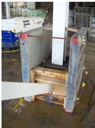
Photograph 9 – Column encasement.
