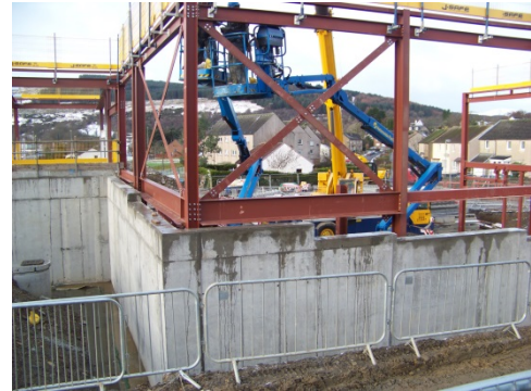
Photograph 6 – Sports Hall steel frame under construction.
